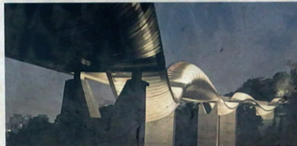
Artfully-placed lights along the bridge create a stunning sight at night.
