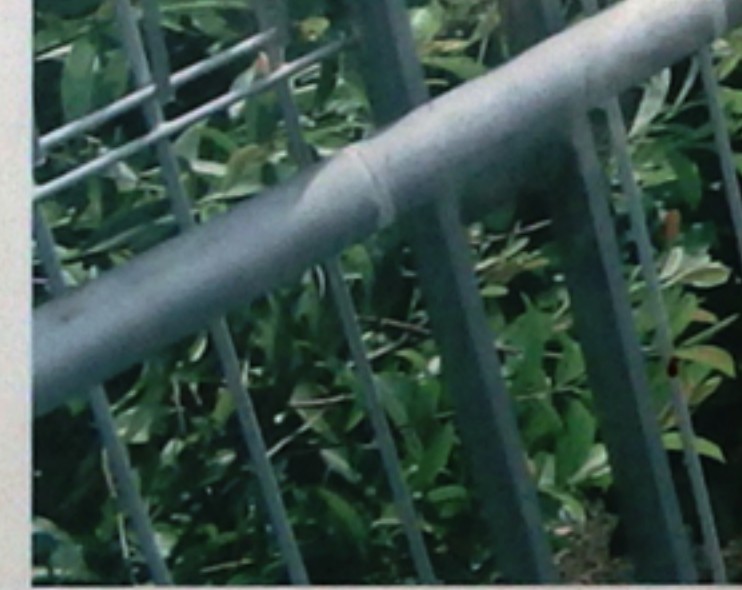
The steps-free elevated walkway zig-zags through steep slopes of hilly terrain.
