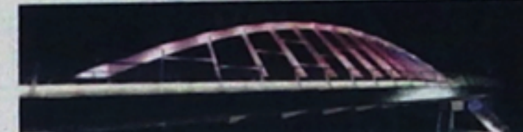
The bridge comes alive at night in the coloured glow of LED lights.
